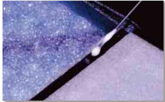
Make sure the hole is filled from the bottom to the top not that just the entry of the hole is filled.
